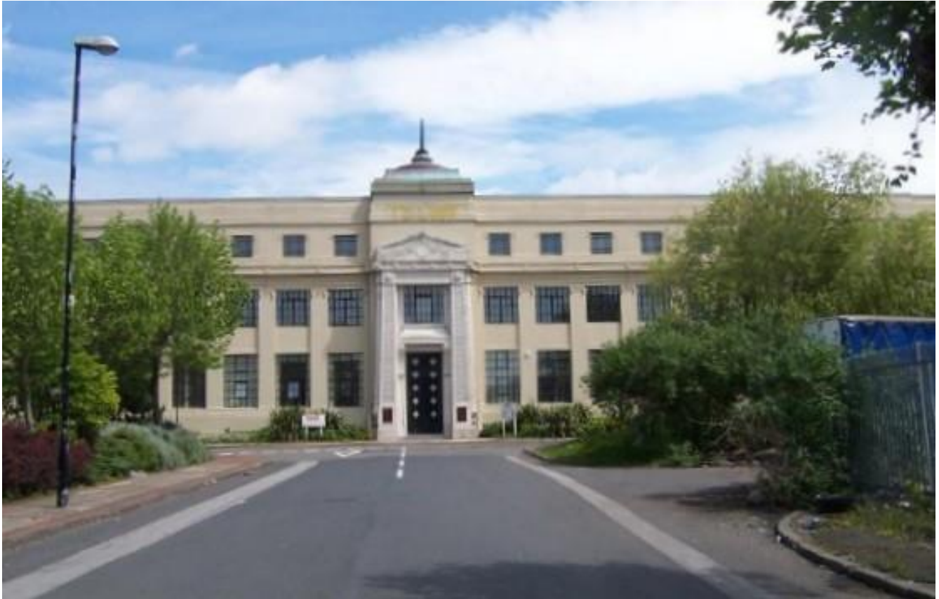
GEC Main Works Administration Block, Witton, Birmingham
