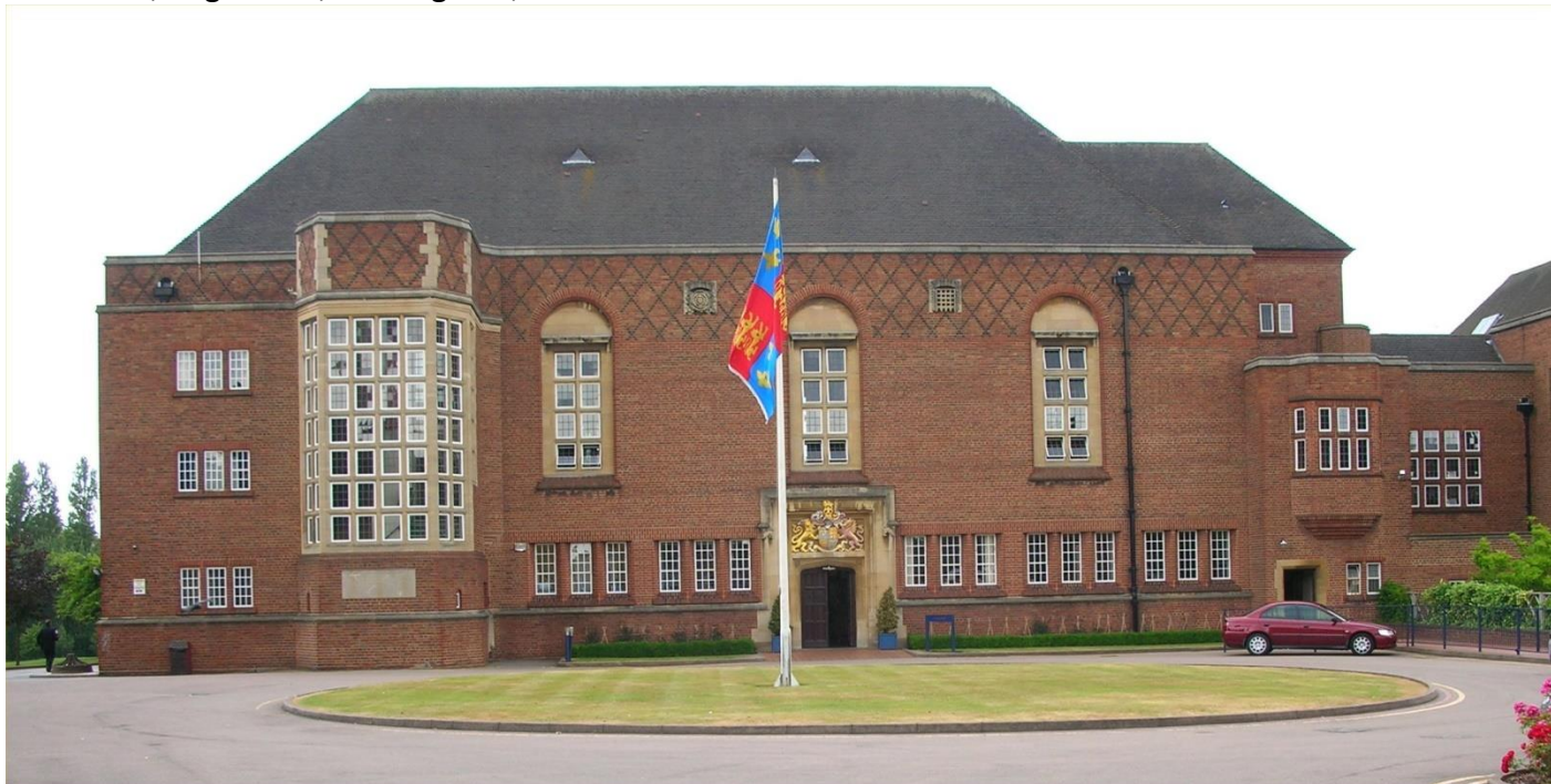
King Edward's School (KES) for Boys in Edgbaston Park Road, Edgbaston, Birmingham, B15.
